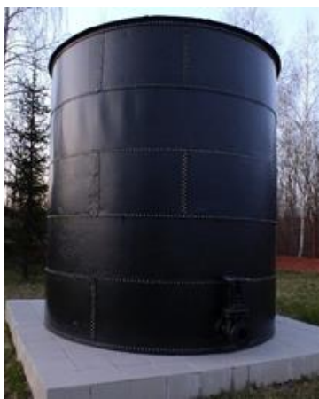
Fig. 6. Oil reservoir, built by Branobel in 1903 with the volume of 119 bbl
